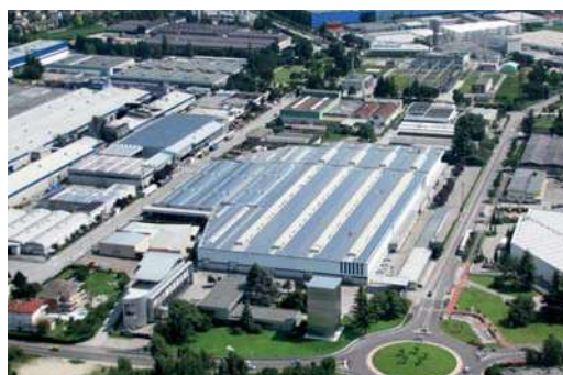
ROVERETO - TN - PREMISES AERIAL VIEW
